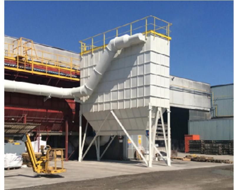
HJL series bag filters are made of carbon steel in thicknesses suited to working with high dust loads for external installation and 24h/day operation.
