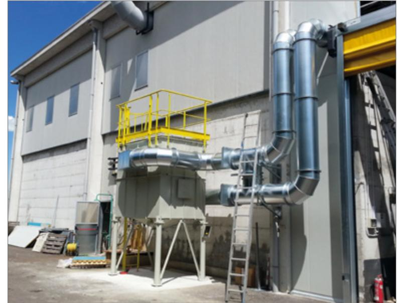
Activated carbon filtration is an air purification technology, thanks to which a gas stream is purified of polluting elements simply going through a bed of active carbons.
