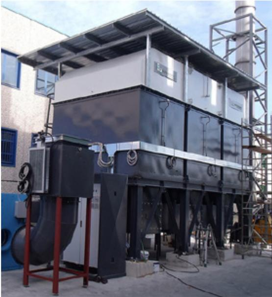
A regenerative thermal oxidizer (RTO) is an abatement system designed to eliminate volatile organic compounds (VOC) and odours from the production lines via incineration.
