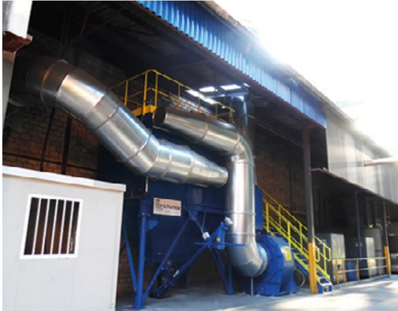
The HJL CART cartridge filter is an equipment used to remove dust from gas streams. The HJL CART could receive as inputs medium/high concentrations of dust, using a very large filtering surface. Thanks to the cartridge features, it's possible to get a large filter surfaces with reduced dimensions.
